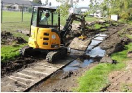
Removal of culvert concrete tops
