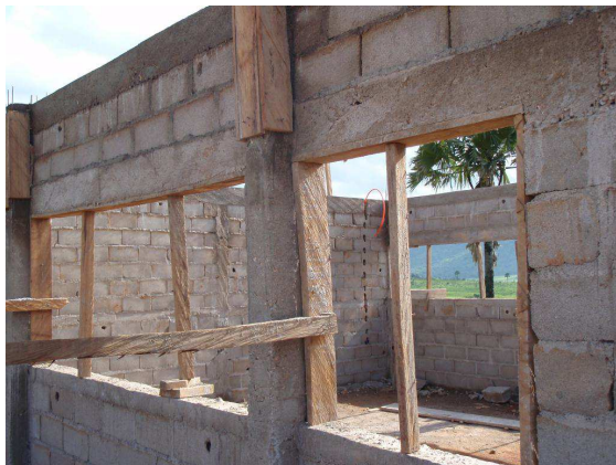
The soon-to-be-completed school at Sambolabo.
