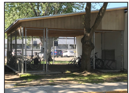
Kelowna's new bike compound is located on campus between the E and H buildings.
