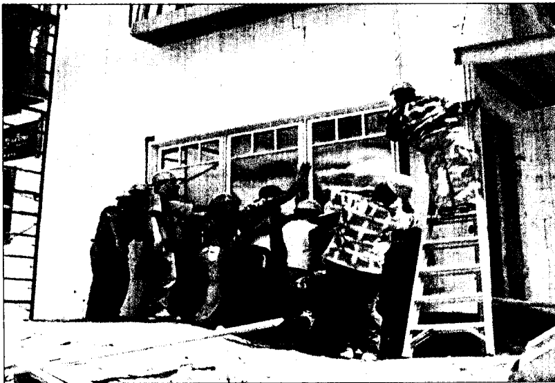
Teamwork helps install All Weather Windows at the Home For Learning
