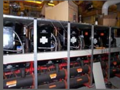
Heat Recovery Chiller - Internal Composition
