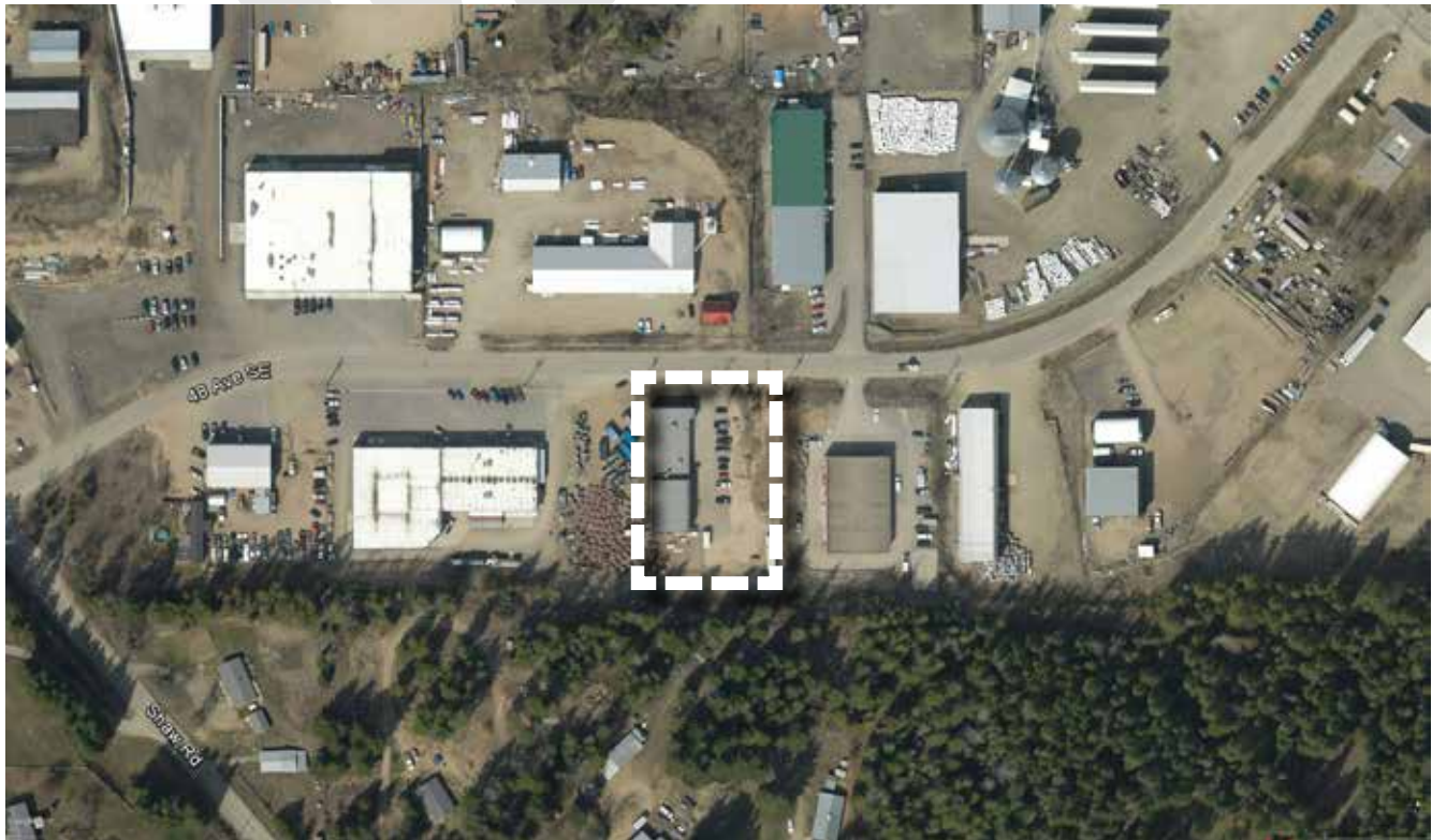
Trades Building and Site
